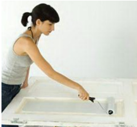
Using a 4" fabric roller (foam does not hold enough paint to work well)
