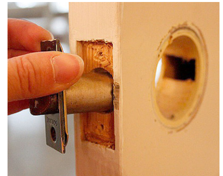
Removing door hardware
